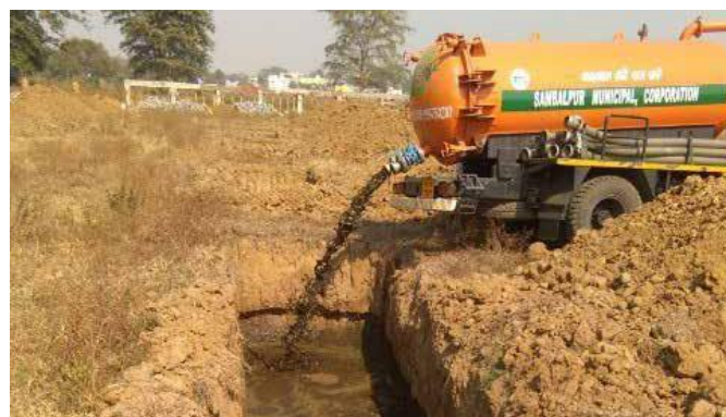
Operators were trained on safe desludging practices
