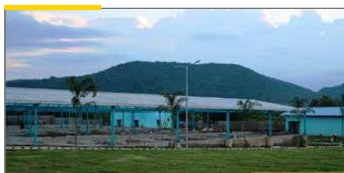
The FSTP other than the tertiary treatment is designed to operate based on gravity model avoiding wear and tear of equipment leading to low operation costs.
