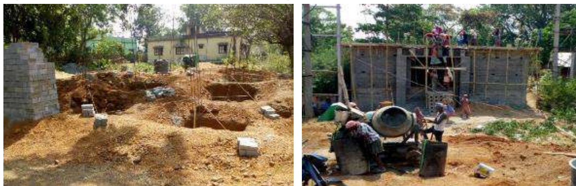
Figure 4-6: Under construction Hybrid toilets at Bugudakata and Murgabadi
