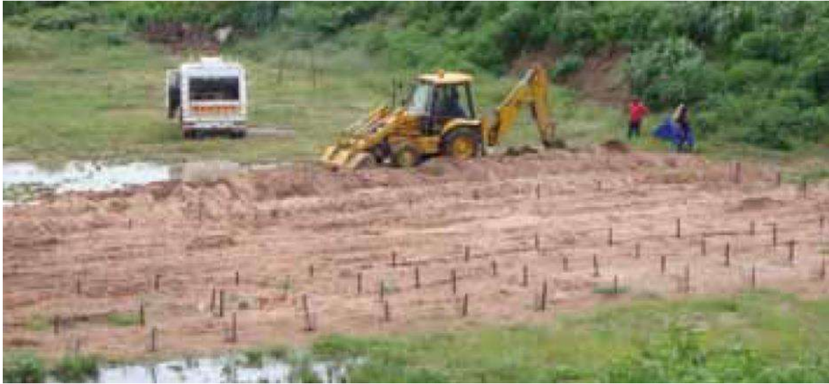
Figure 4-10: -Typical deep row entrenchment site
