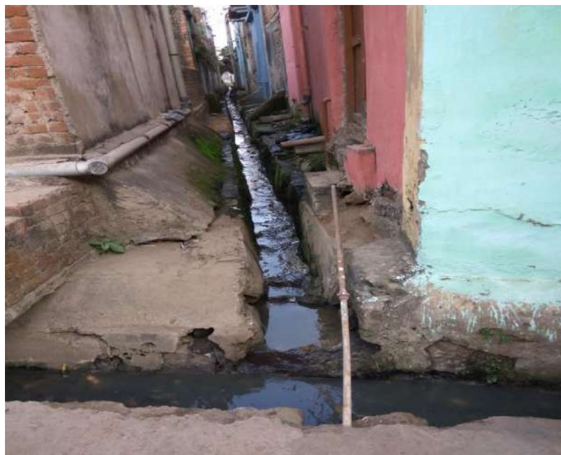
Figure 2-4: -Insanitary toilet directly connected to open drains
