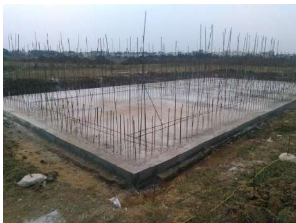
Figure 4-9: -On-going work at Berhampur SeTP
