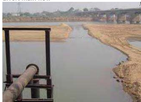
Figure 2-6: -Intake pipes on Kuakhai River - Picture showing channel dug on riverbed to divert main flow
