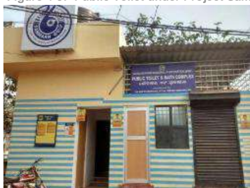
Figure 4-5: -Public Toilet under Project Samman at Bapuji Nagar, Ward No. 53
