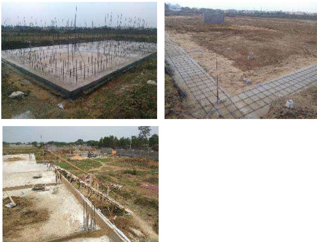
Figure 4-18: -On-going work at Bhubaneswar SeTP (co-treatment within STP)
