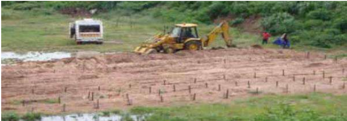
Figure 4-19: -Typical deep row entrenchment site
