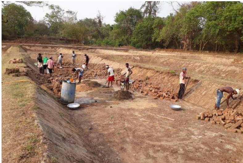
Figure 4-14: -On-going work at Cuttack SeTP (co-treatment within STP)
