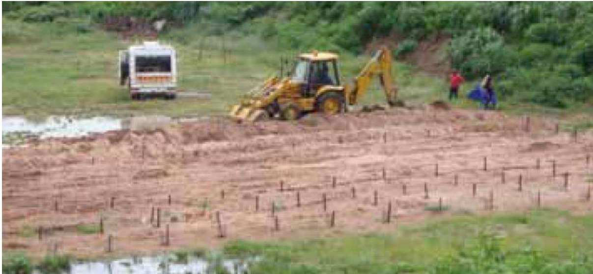
Figure 4-15: -Typical deep row entrenchment site
