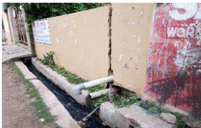
Figure 4-3: - Toilet outlet into open drain
